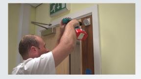
Align the keeper plate with the magnet face.
