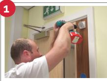
The Agrippa door holder is battery powered and wire-free. The device is installed at the top of the door and is pre-progammed to work.
