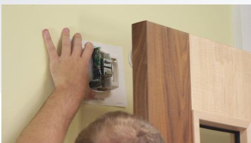
Use the paper template supplied to drill holes in the wall (remember to wear personal protective equipment (PPE) and check for wires!)
