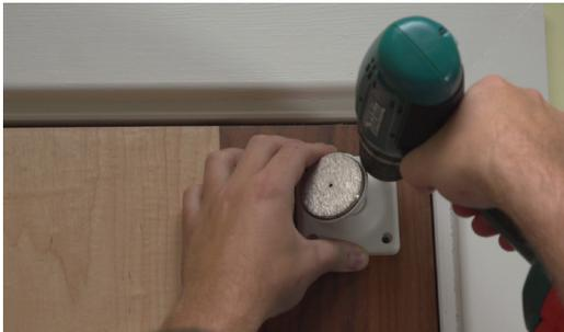
Check the rubber ring is fitted before screwing the keeper plate to the door.
