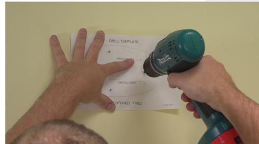
Remove the lid and fit the holder securely to the wall using three screws.
