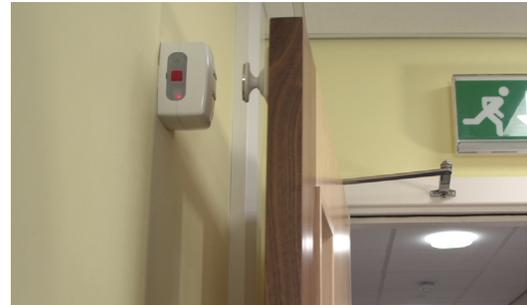
The holder takes another two minutes to process the sound. This is indicated by the rotating pattern on the display.
